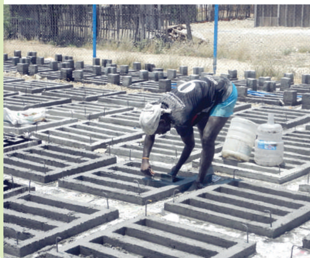
Construction of concrete frames
