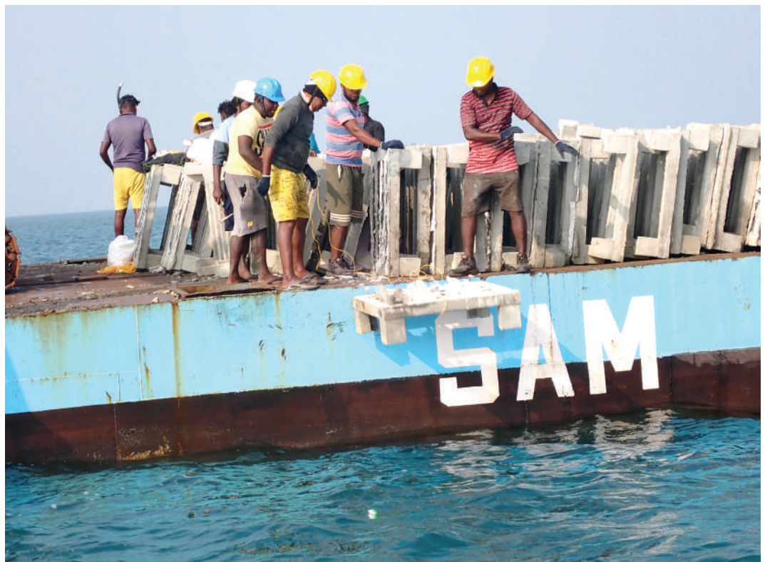
Deployment of substrates in the restoration site
