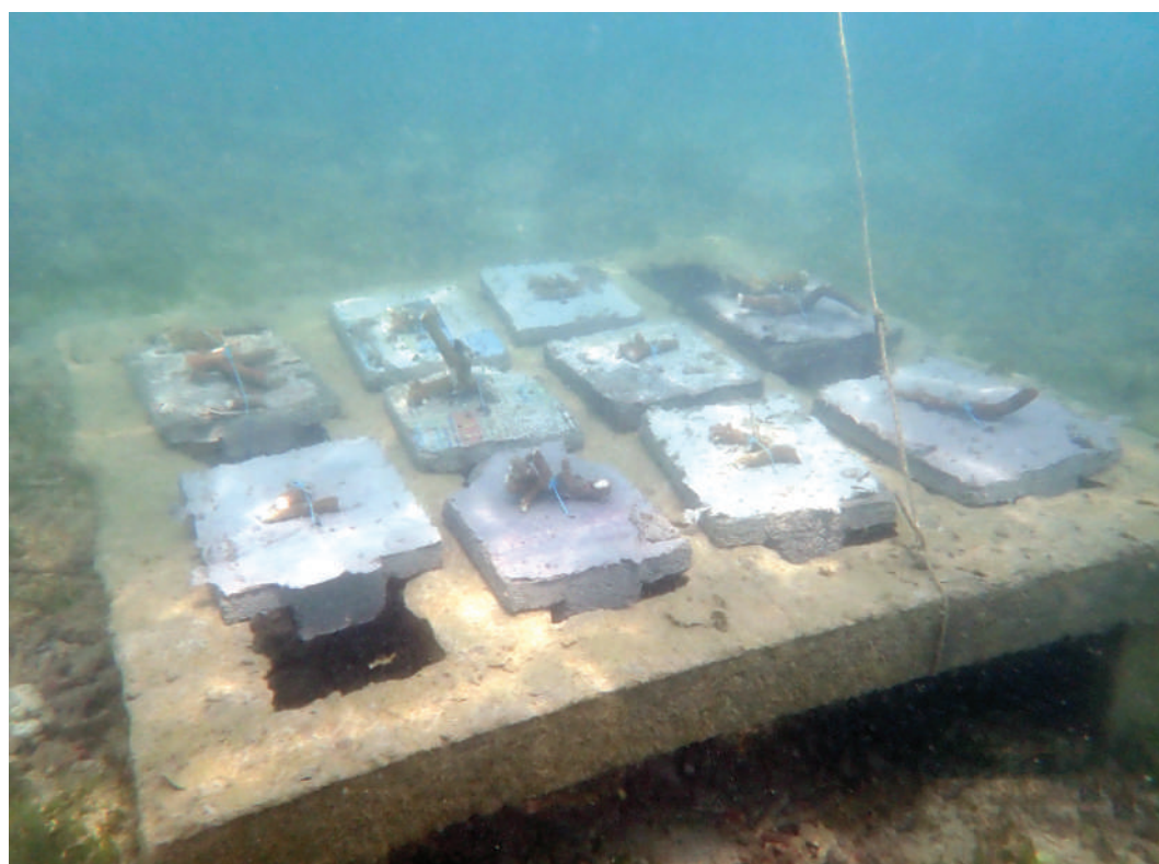
Underwater fixing of cement slabs
